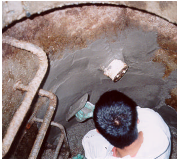
Figure 2. – Trowel application of patching material in manhole on Marine Drive (August 2001). Photo by Jon Walter
